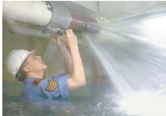
Sea Cadet Stephen Terrill fits a jubilee patch onto a ruptured fire main Friday during damage control training. (David Hansen/Daily News staff)
